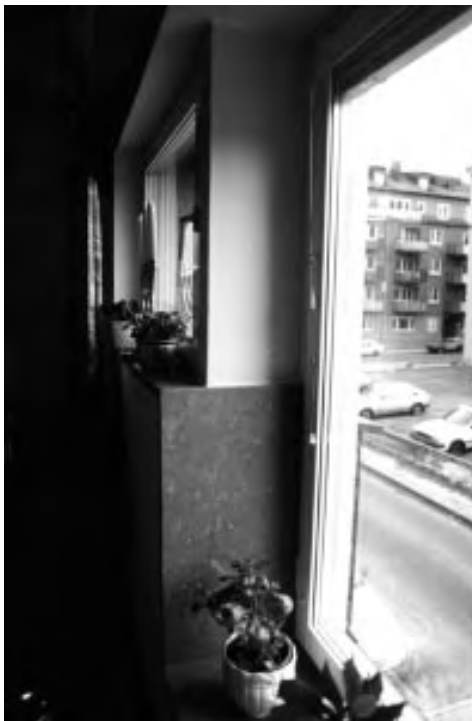
Bay window, detail.
