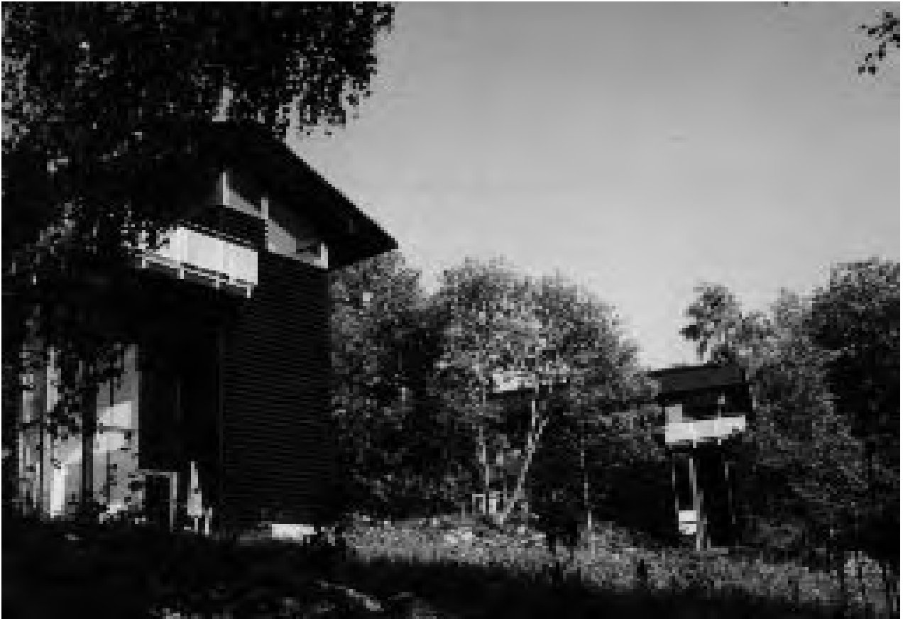
The Nielsen block of the Hestra housing development. The southern group of buildings.
