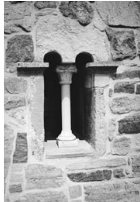
Muntin bars modulate the effect of a hole in the wall and accentuate the enclosing wall's sheltering capacity.
