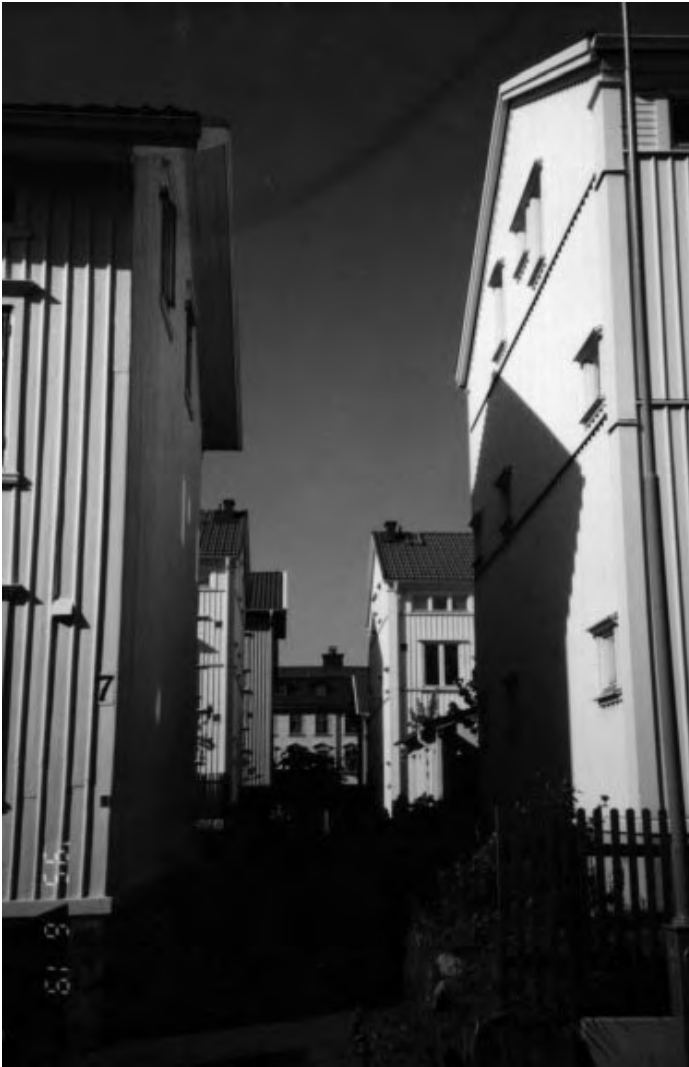
View of both of the newly built blocks.
