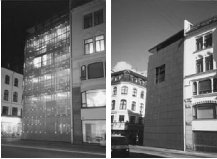
The BT building, Copenhagen. Architect: Henning Larsen, 1994. Night and day photographs. A screen of perforated steel gives the façade different characteristics by day and by night.
