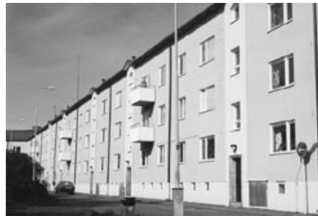
Façade facing courtyard.
