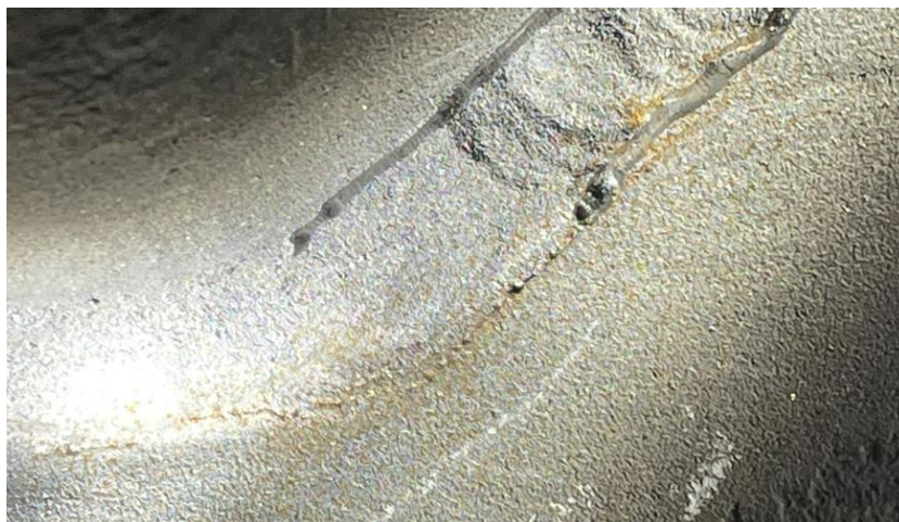
Figure 10: HFMI-treatment revealing shallow, sub-surface porosity. Also visible are surface (possibly cold) cracks at weld toe. Such weld should be repaired prior to HFMI-treatment.
