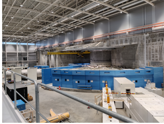
(c) ESS (under construction)
