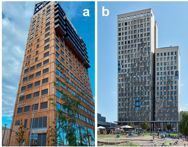
Figure 12.2 (a) Mjøstårnet, Norway. At 84.5 metres, it is currently one of the world's tallest timber buildings (photo Peter Lang, Rothoblaas). (b) HoHo in Austria (photo proHolz Austria / Bruno Klomfar).
