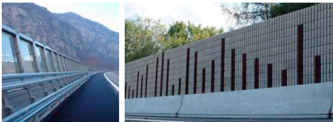
Fig. 2. Different types of integrated noise and safety barriers of different materials in Europe (steel & transparent left side and fully concrete type right side).
