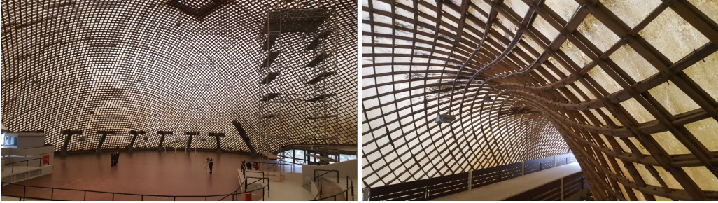
Figure 1.1: Timber grid shell in Mannheim (1975) by Frei Otto (1925-2015) together with structural engineers Ted Happold (1930 – 1996), Ian Liddell and Chris Williams from Structures Group 3 at Arup.
