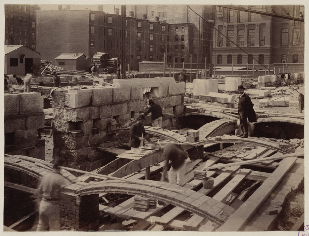
Figure 4.10: Master builder Rafael Guastavino Sr. standing on a recently finished arch during the construction of the Boston Public Library, 1889.
