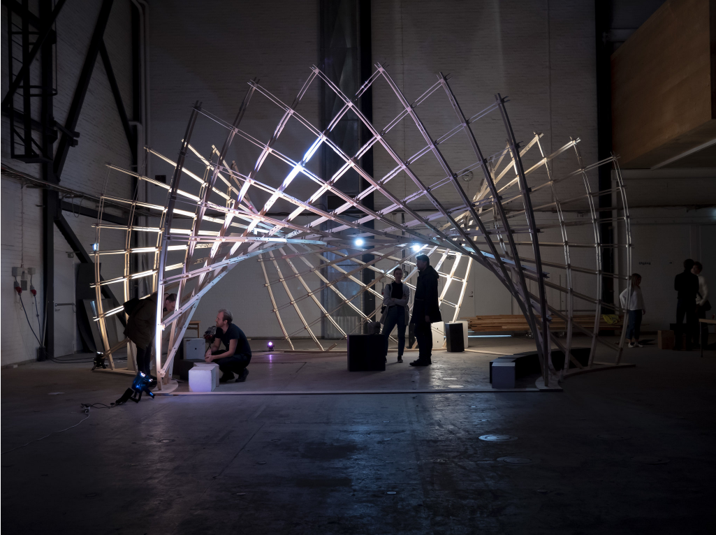
Figure 2: The exhibition of the asymptotic timber grid shell built during the 2019 workshop.
