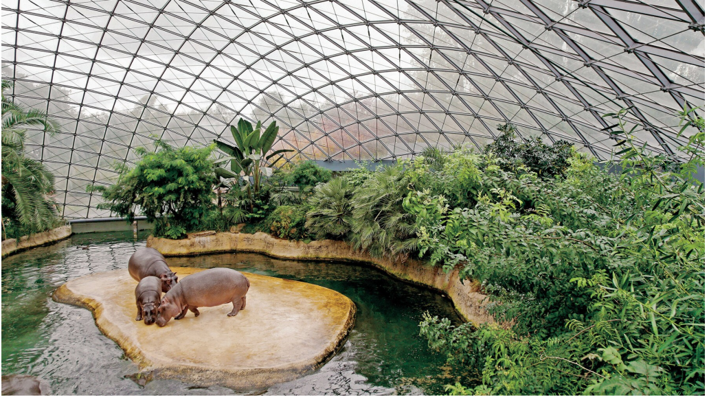
Figure 4.12: Steel grid shell at the House for Hippopotamus at Berlin Zoo was designed such that it could be covered by planar quad panels. Schlaich Bergermann Partner, 1996.
