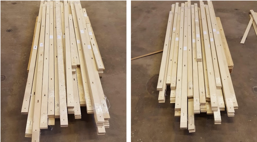
Figure A.25: The grid shell was disassembled after the workshop, and the timber laths were grouped together and could easily fit on two pallets for storage and possible reuse.
