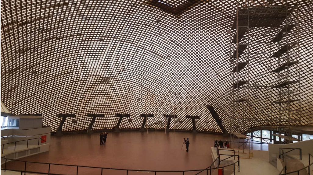
Figure 4.13: Timber grid shell in Mannheim (1975) by Frei Otto (1925-2015) together with structural engineers Ted Happold (1930 – 1996), Ian Liddell and Chris Williams from Structures Group 3 at Arup.
