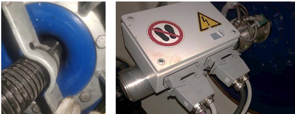
Figure 3.7: Hub power cable through hollow shaft hub side view and nacelle side view with the slipping connection box.
