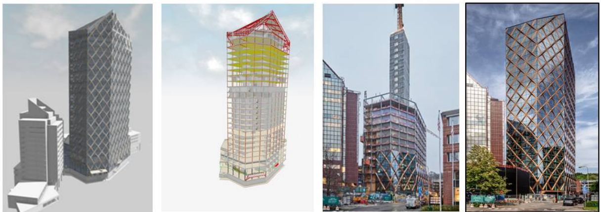
Fig. 10: The Kinum project; BIM, structural-only BIM, construction, completed building (left to right).
