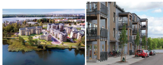
Figure 7: Arken (CLT 4) constructed in CLT in Växjö, Sweden
