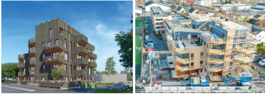
Figure 3: St. Olavsvei 18 project (CLT 3) constructed with CLT in Kristiansand, Norway
