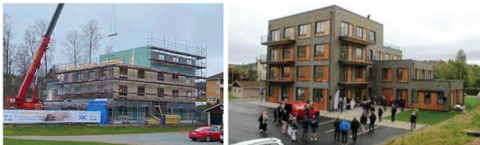
Figure 8: Björkdungen 5 (CLT 5) constructed in CLT in Bengtsfors, Sweden
