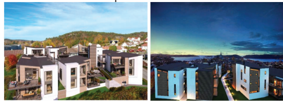
Figure 6: Fagertun Panorama (Concrete 3) constructed in concrete in Lillesand, Norway
