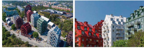
Figure 9: Tingstorget (Concrete 3) constructed in concrete in Botkyrka, Sweden
