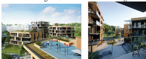
Figure 5: Trelasttomta (Concrete 2) constructed in concrete in Myrvoll, Norway
