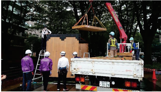
(f) Construction of the roofs
