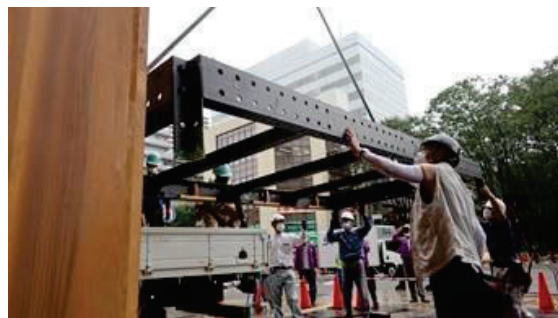
(e) Construction of the steel beam frame
