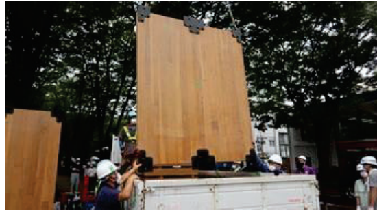
(c) Installation of the CLT walls
