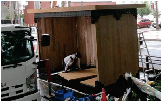
(g) Construction of the floors
