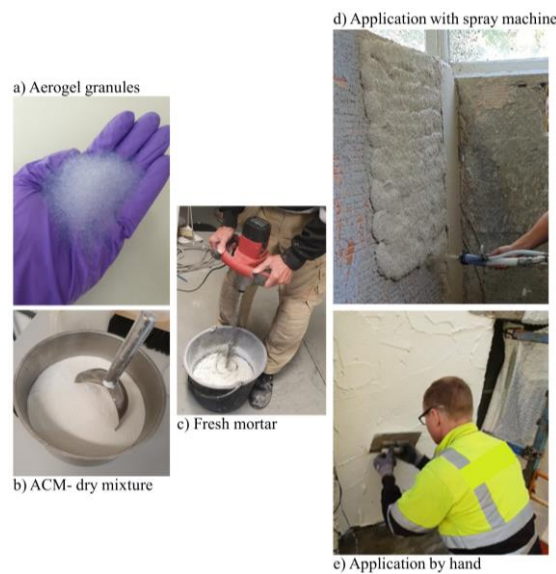
Figure 2. a) Aerogel granules. b) Dry mixture of ACM. c) Preparation of fresh mortar by blending the ACM with water. d) Application with spray machine. e) Application by hand.
