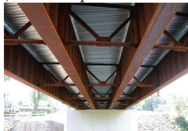
(b) Girder bridge, Demonstration bridge in Bradford County, PA, USA [21]
