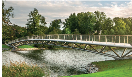
(b) Folke Bernadotte bridge, photo courtesy of Stål and Rörmontage [11]
