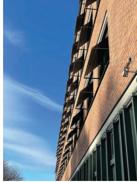
Figure 11.75 Photo of the A-building's exterior screens.
