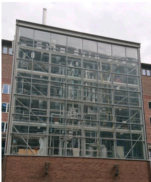
Fig. 3. Pilot evaporator used in this work.
