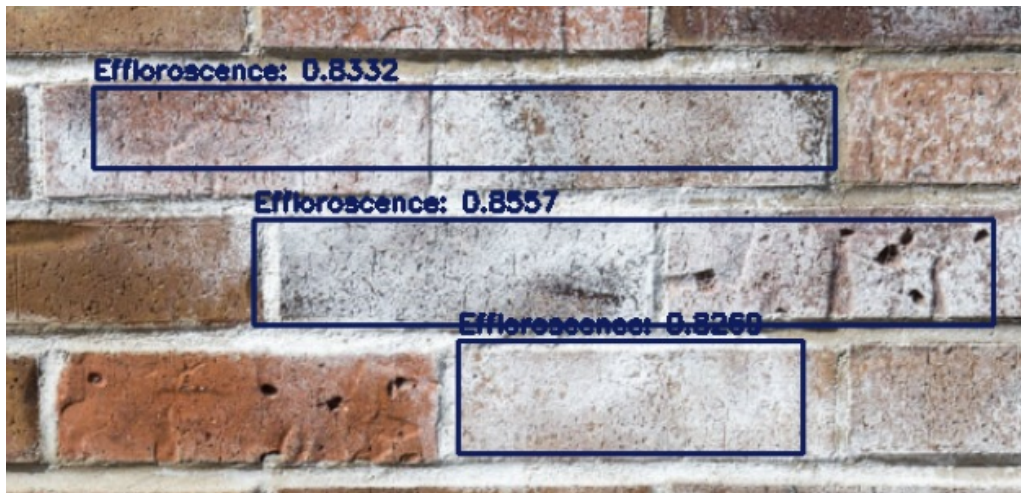
FIGURE 1. Example of output from the Build-Sense model – model draw bounding boxes around damaged area alongside with its level of confidence [18].
