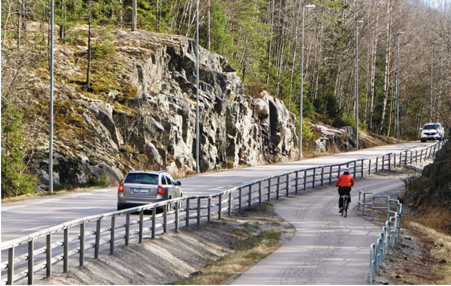
Fig. 4 Example of how vulnerable road users could be separated from motor vehicles on rural roads. (Photo: Anders Kullgren)
