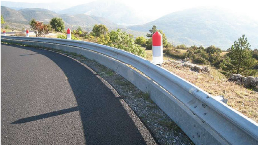
Fig. 11 Example of W-beam barrier with an added MPS. Photo: SMC, Sweden
