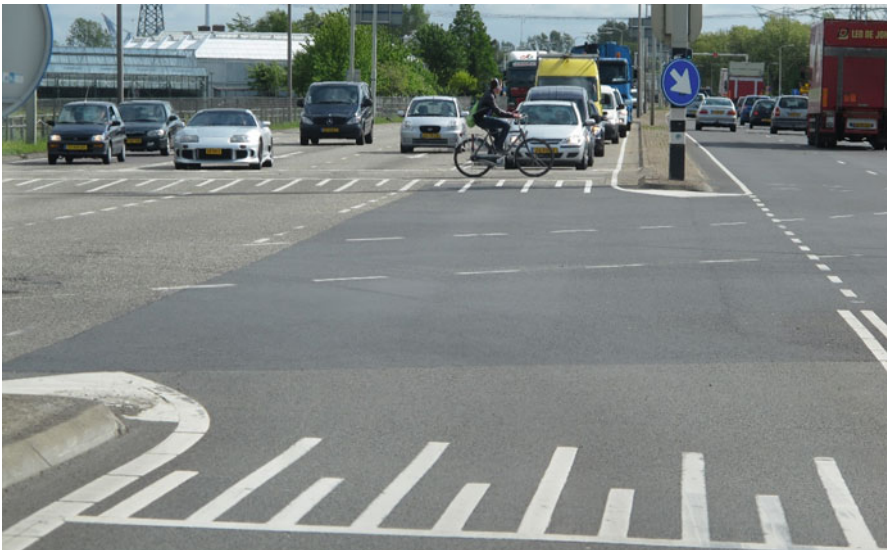
Fig. 14 Urban signalized intersection with speed platforms for cyclists and pedestrians (The Netherlands)
