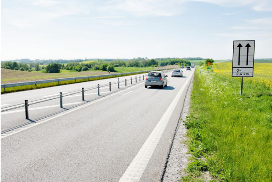
Fig. 10 Example of a design of a 2 + 1 lane road. Photo: The Swedish Transport Administration
