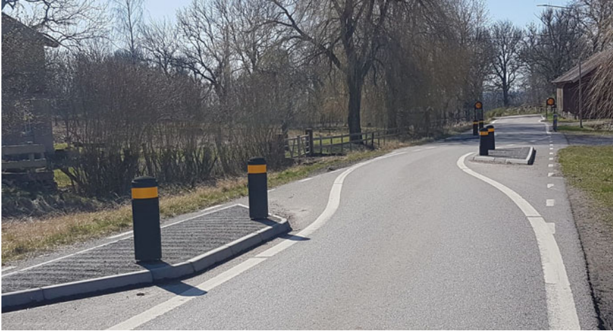
Fig. 3 Example of use of a chicane to control vehicle speed. Photo: Helena Stigson
