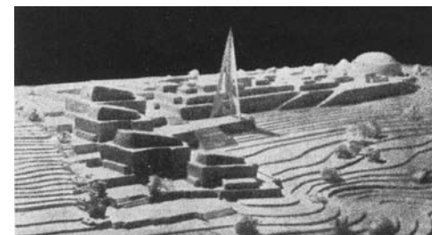
FIG. 6: Jørn Utzon. Crystal Palace competition in London, 1947. The entry arranged the main auditorium and fourth performance halls and exhibition spaces on a terraced platform which frames the perimeter of the site.
