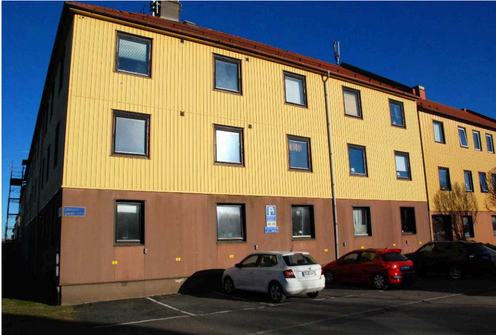
Example of an insensitive 1970s energy retrofit of working-class housing, Gothenburg (Sweden), 2017. © Paula Femenias.
