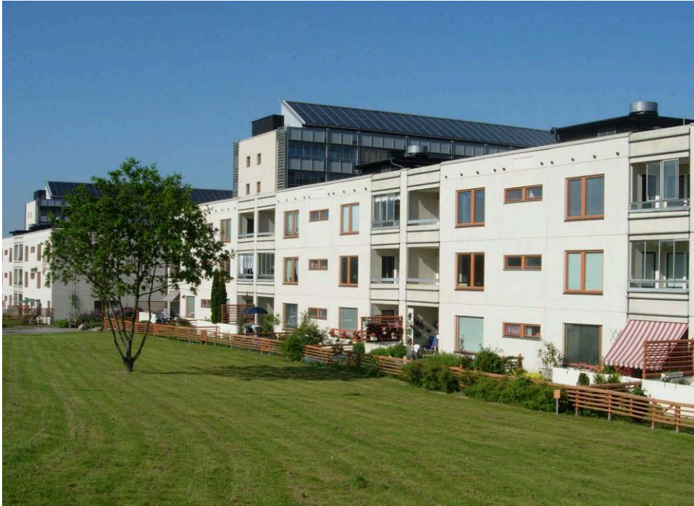
Solar Houses in Västra Gårdsten after renovation, in the back the high-rise blocks with solar panels on the roof, Västra Gårdsten, Gothenburg (Sweden), 2016.
