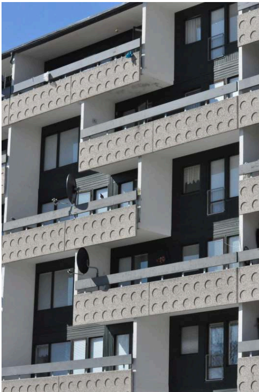
Details of the façade and the reconstructed balcony fronts, Skolspåret (Sweden), 2021.
