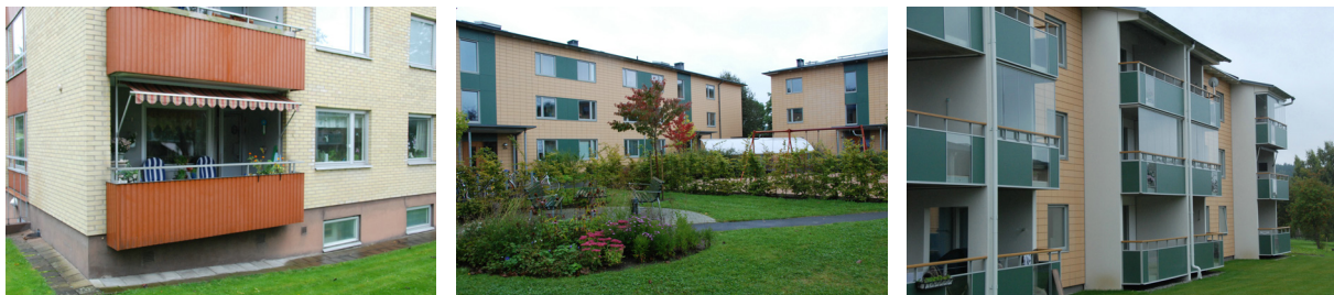
Figure 3 Case C before the renovation (left) and after (middle and right), showing the final design of the balconies.
