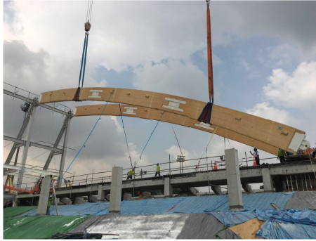
(a) Arch with moment resisting joints during construction © Ermanno Acler [24]
