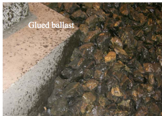
Figure 6. Glued ballast [55]
