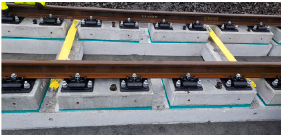
Fig. 5. A view of the 3 MB slab design consisting of base slabs, top blocks, and an elastomeric layer between the concrete layers.
