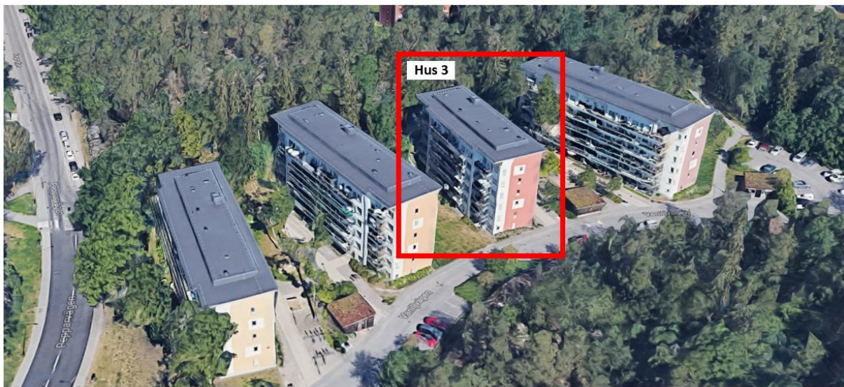
Figure 1. General view of the Blå Jungfrun building complex. The reference building (hus 3) is highlighted. Source: https://www.google.se/maps/@59.2499423,18.0908937,111a,35y,306.19h,61.72t/data=!3m1!1e3?hl=sv
