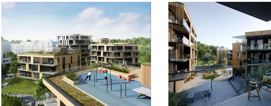
Figure 6 - Trelasttomta (Concrete 2) constructed in concrete in Myrvoll, Norway
