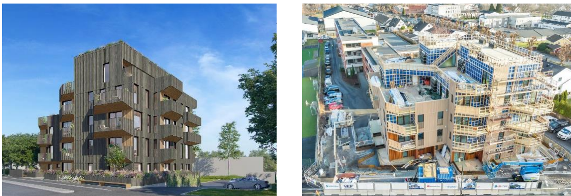
Figure 4 - St. Olavsvej 18 project (CLT 3) constructed with CLT in Kristiansand, Norway
