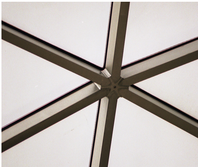
Figure 2.19: Flame cut star-shaped node of the Great Court roof for the British Museum in London. The nodes were attached to the rectangular members using welding on site. See attribution in the figure credits list.
