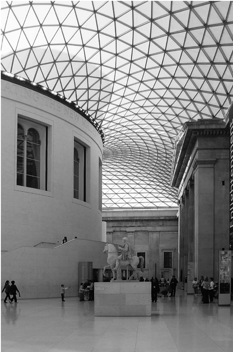
Figure 2.39: The great court roof structure at the British museum deigned by Chris Williams. The shape is defined such that the horizontal thrust is concentrated to the corners. The project was an important reference for the work with the Mexico City Airport project. See attribution in figure credits list.
