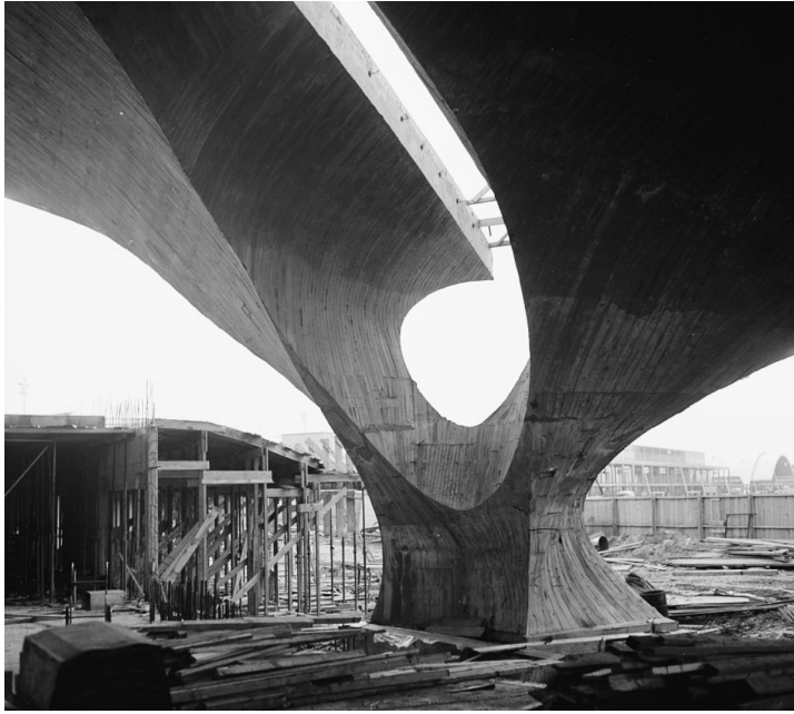
Figure 2.24: A photo from the construction of the TWA terminal in New York City in the early 1960s. The in-situ concrete joint is characterised by the seem less blending of roof and column. See attribution in the figure credits list.
