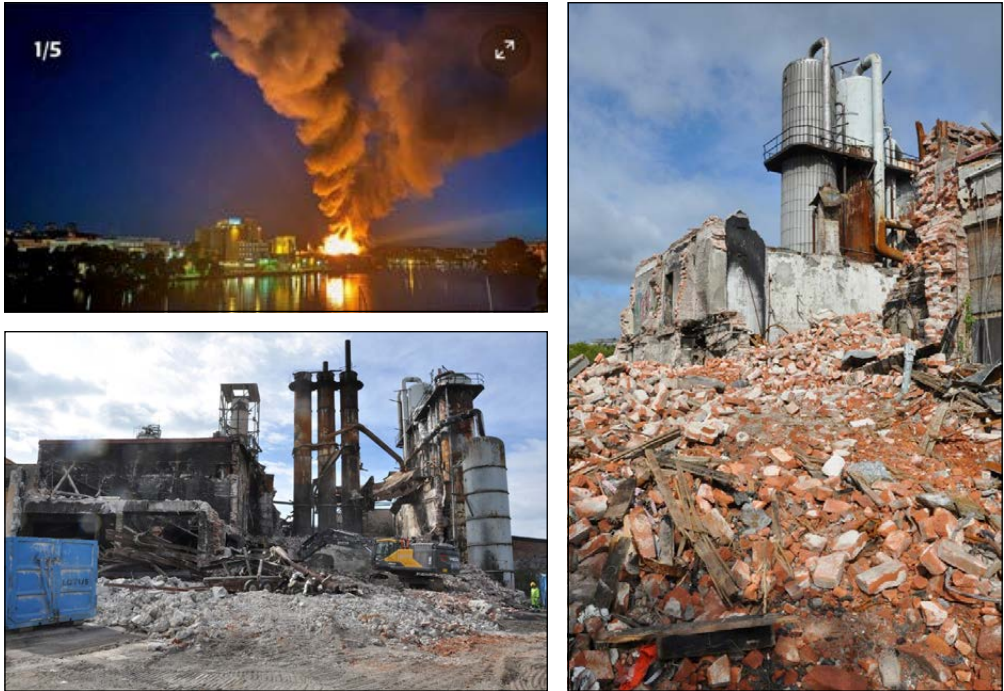
Figure 21 a-c. The former Carbonic Acid Factory at Lövholmen (21a top left) caught fire on 29th of July 2021. Source: The newspaper Svenska Dagbladet (SvD) 2021-07-30. After securing the premises, a ruin with heaps of brick, concrete rubble, reinforcing bars and cisterns is what is left of Kolsyrefabriken (21b top right and 21c above). Photographs Nyréns, Urban Nilsson 2021-09-01
