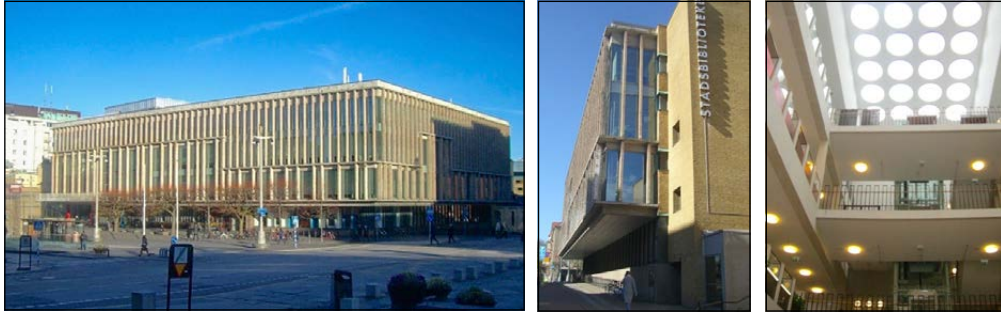
Figure 9, 10 and 11. The original facade seen from inside. To the left, the brick façade seen in the corridor at the ground floor. In the middle the café in the extension at the second floor seen from the third floor. To the right, stairs to the third floor. Photography: Magnus Rönn, 2020.
