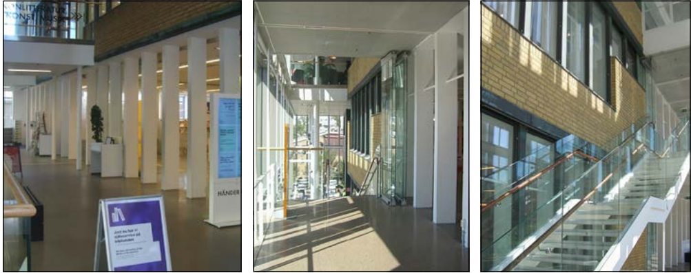
Figure 6, 7 and 8. The original facade seen from inside. To the left, the brick façade seen in the corridor at the ground floor. In the middle the café in the extension at the second floor seen from the third floor. To the right, stairs to the third floor. Photography: Magnus Rönn, 2020.
