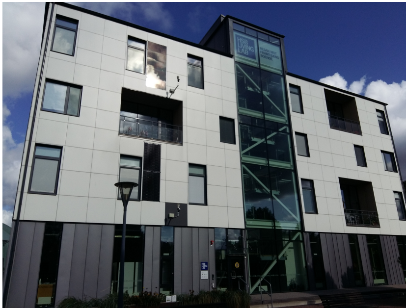
Figure 3.6: The facade of the HSB LL building.
