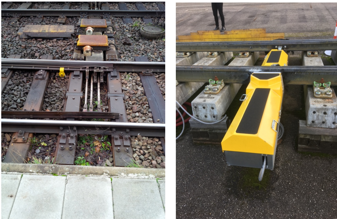
Figure 22 Two types of drives: To the left a traditional design with open bar installation, and to the right a modern design with built-in bars of the type Easyswitch. Picture courtesy A Alqvist, Vossloh.
