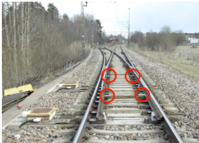
Figure 4 Picture of a switch with four TKKs. Picture courtesy Jan-Erik Meyer, Trafikverket.
