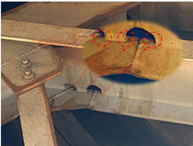
Fig. 9 Examples on cope holes in a welded steel bridge
