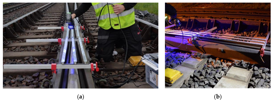
Figure 2. (a,b) The 3D geometry scan of a crossing transition with Creaform HandySCAN 3D laser scanner [19].
