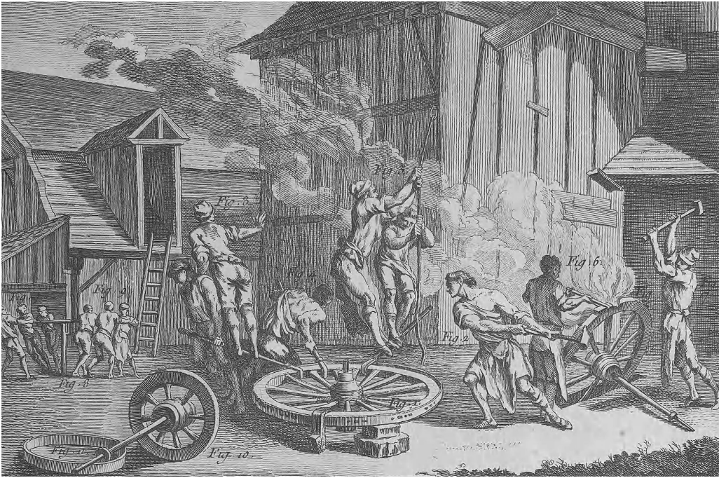
Figure 2.14: Two methods of shoeing a wheel. In the centre the labourers are using hammers and ‘devils’ to fit a hoop onto the rim, and on the right they’re hammering strakes into place.
