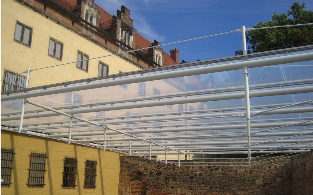
Figure 2.18: Lutherhaus, Germany (2010). Pressurised transparent foil cushions suspended between cable-supported steel beams.
