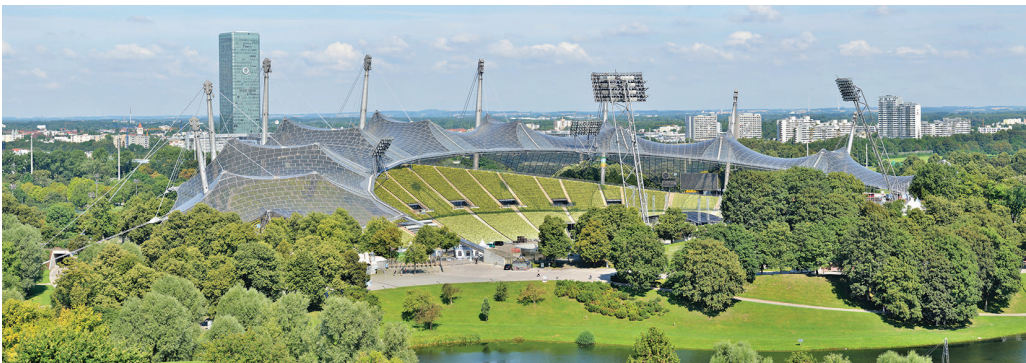
Figure 2.20: Olympiastadion (1972) in Munich by Frei Otto, Jörg Schlaich, Rudolf Bergermann, et al
