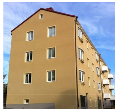
Figure 6. Company B, building in same area as Fig. 5 after external insulation, new plaster and windows. Photo: L. Thuvander
