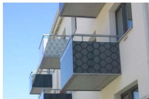
Figure 4. Company A, a 1950s area where façade, balconies and windows have been altered in a recent renovation. Photo: L. Thuvander
