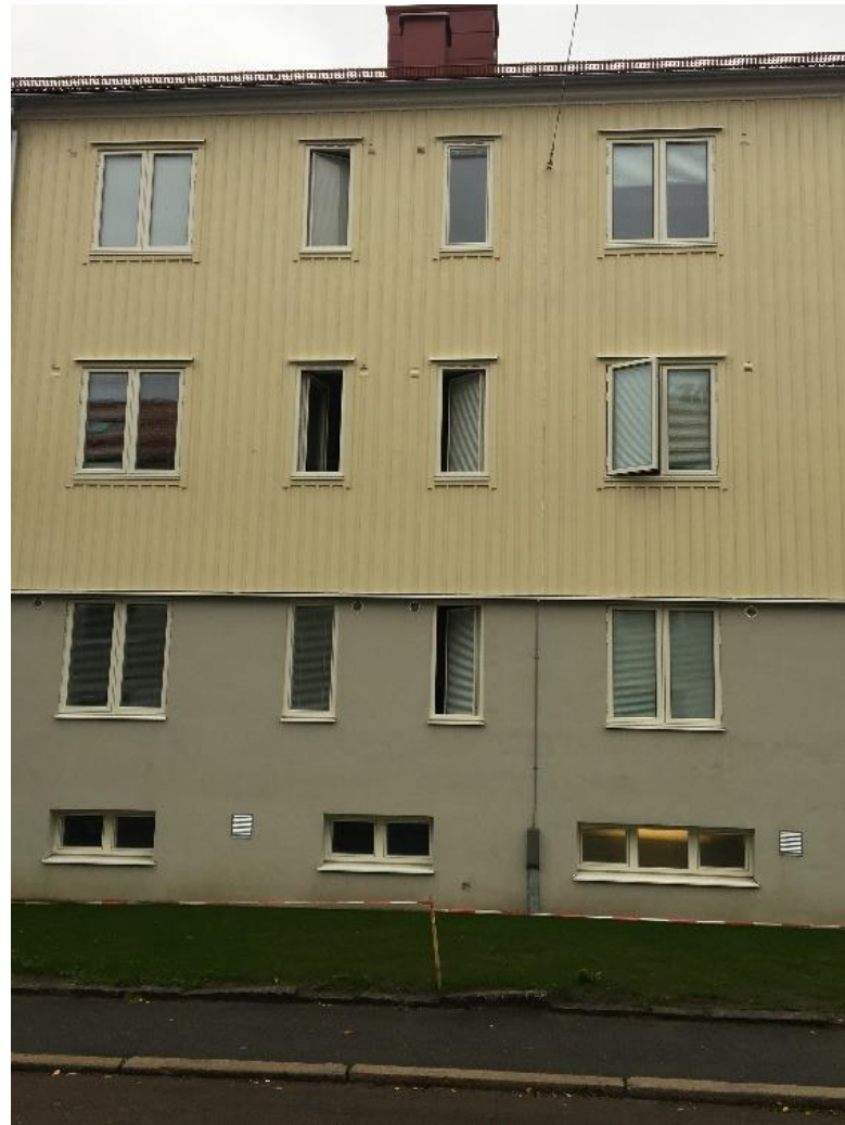
Figure 8. Side-hinged windows in a new phase of renovations in the area, which to a higher degree resemble the original windows and façades. Photo P. Femenias 2018.
