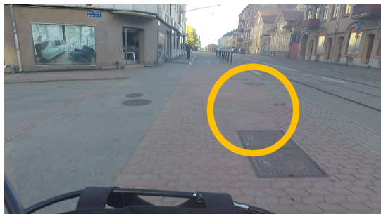
Figure 2a. The rugged maintenance holes on the ground to the right acts as obstacles for cyclists. The cyclists travels to the left.
