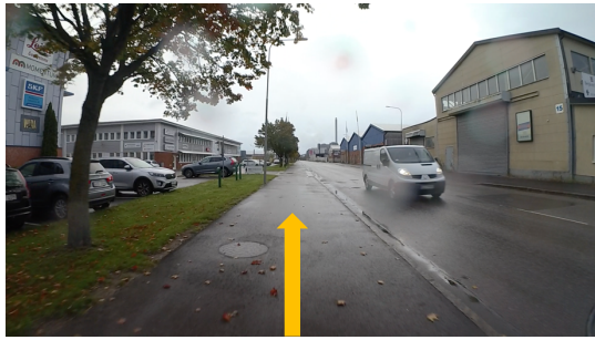
Figure 6a. The lane edge to the right acts as an insufficient divider. Cyclists travel in the middle of lane.
