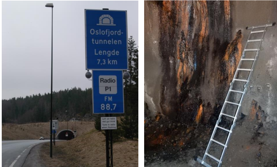
Figure 7. The Oslofjord tunnel entrance (left) and microbial biofilm material on sprayed concrete on the tunnel wall (right).
