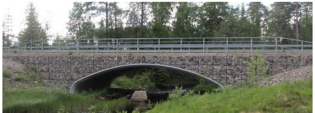
Figure 5. Box culvert bridge over Siktån in Rörbäcksnäs [5].
