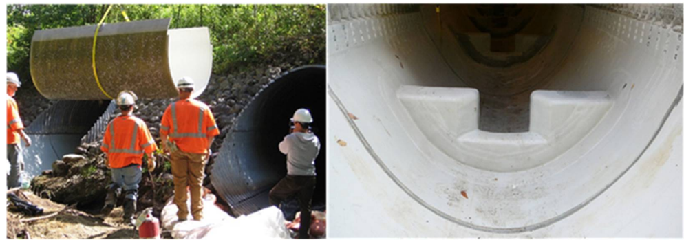
Figure 3. Refurbishment of a corroded steel culvert using partial FRP lining [21].
