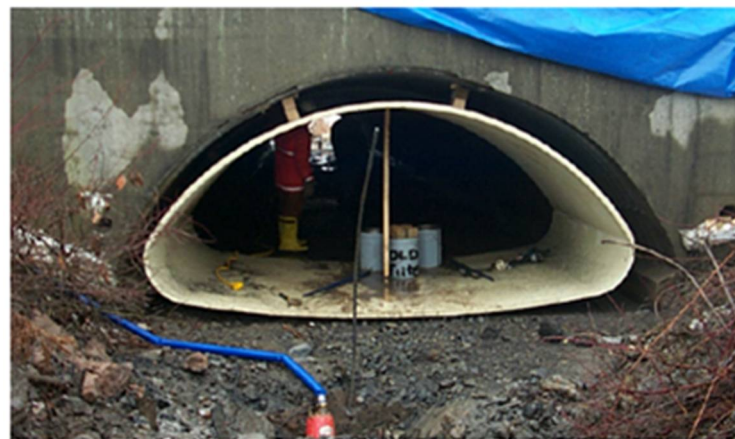
Figure 4. An entire culvert re-lining in Buffalo (USA) using FRP [22].
