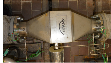
Fig. 3. Exhaust evaporator.
