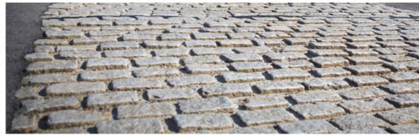
Figure 6: Belgian pave road surface [71].
