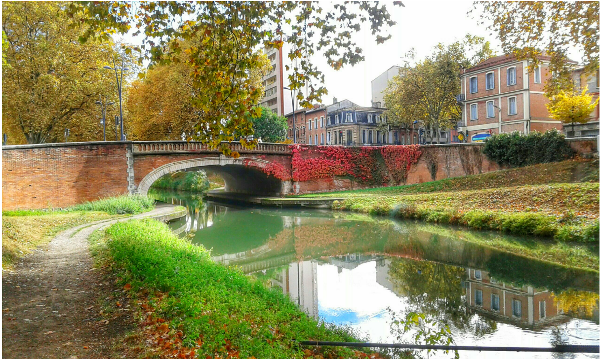
Figure 5: Pont de l' Avenue by Paul Séjourné over the Canal de Brienne in Toulouse. Photo by Cesar Sabas licensed under CC BY-SA 4.0, https://commons.wikimedia.org/w/index.php?curid=44584947
