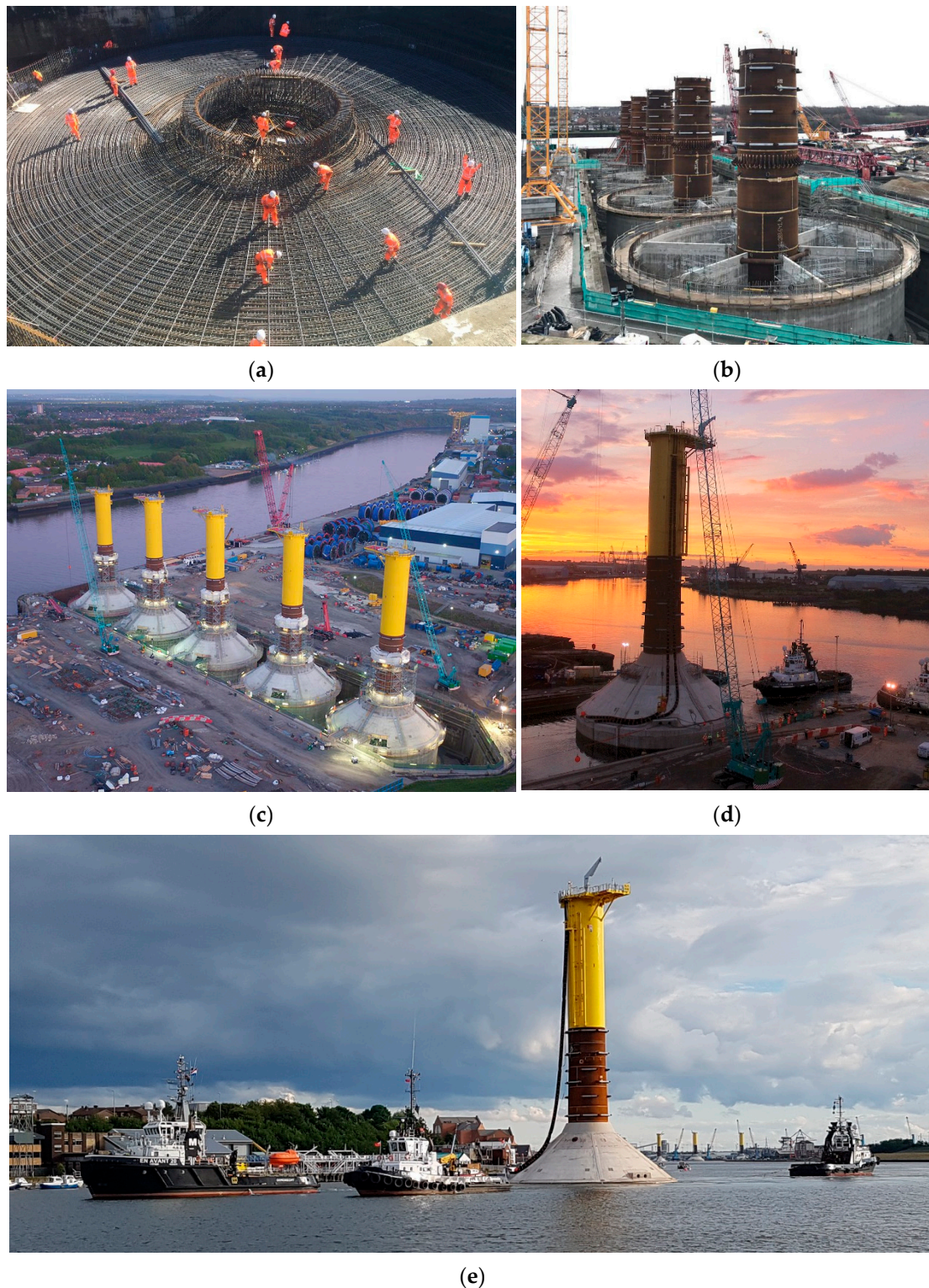
Figure 12. Construction of gravity-based concrete substructures for the Blyth Offshore Demonstrator Project: (a) reinforcement placing, (b,c) construction of the concrete base and steel shaft of the substructures in the dry dock, (d,e) transport of the self-floating substructures using tugboats. Credit: BAM Nuttall, reproduced with permission.
