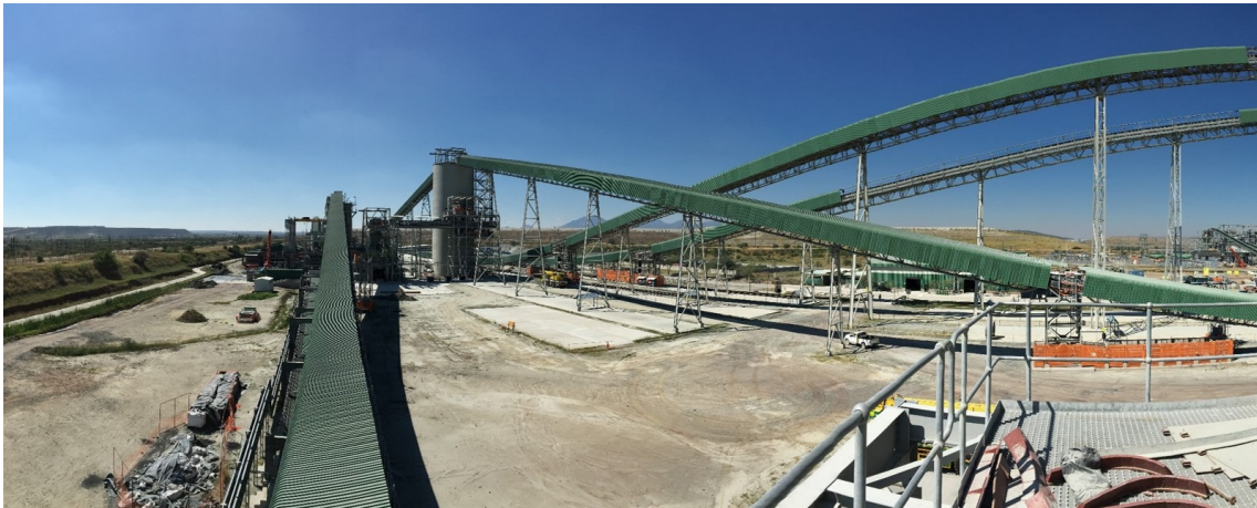
Figure 1.2: A minerals processing plant and an overview of the conveying system between crushers, screens and storage units.
