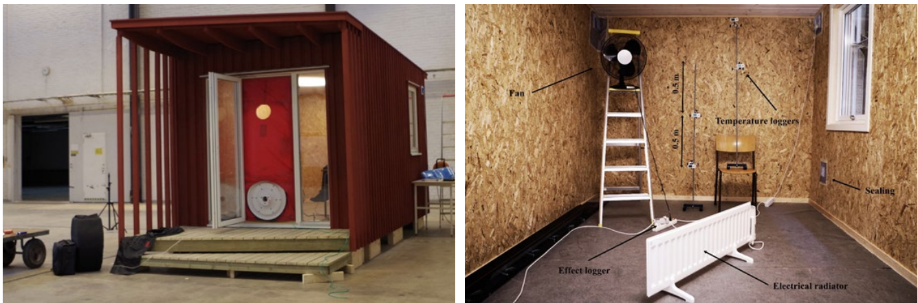
Figure 3 To the left: the summer cottage from the outside, during a blower door test. To the right: the interior of the summer cottage during the co-heating test.
