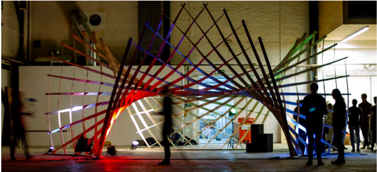
Figure 1: The asymptotic gridshell built during two days in the workshop in December 2018 by the students based on design provided by the workshop leaders, photo: Martin Skarby.
