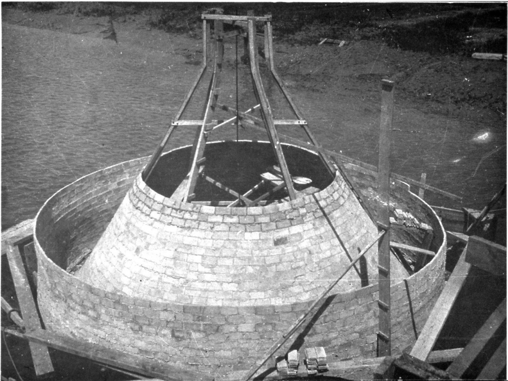
Figure 2.17: Eduardo Torroja using thin brick shells as form-work for the foundations of the Sancti Petri Bridge, 1927
