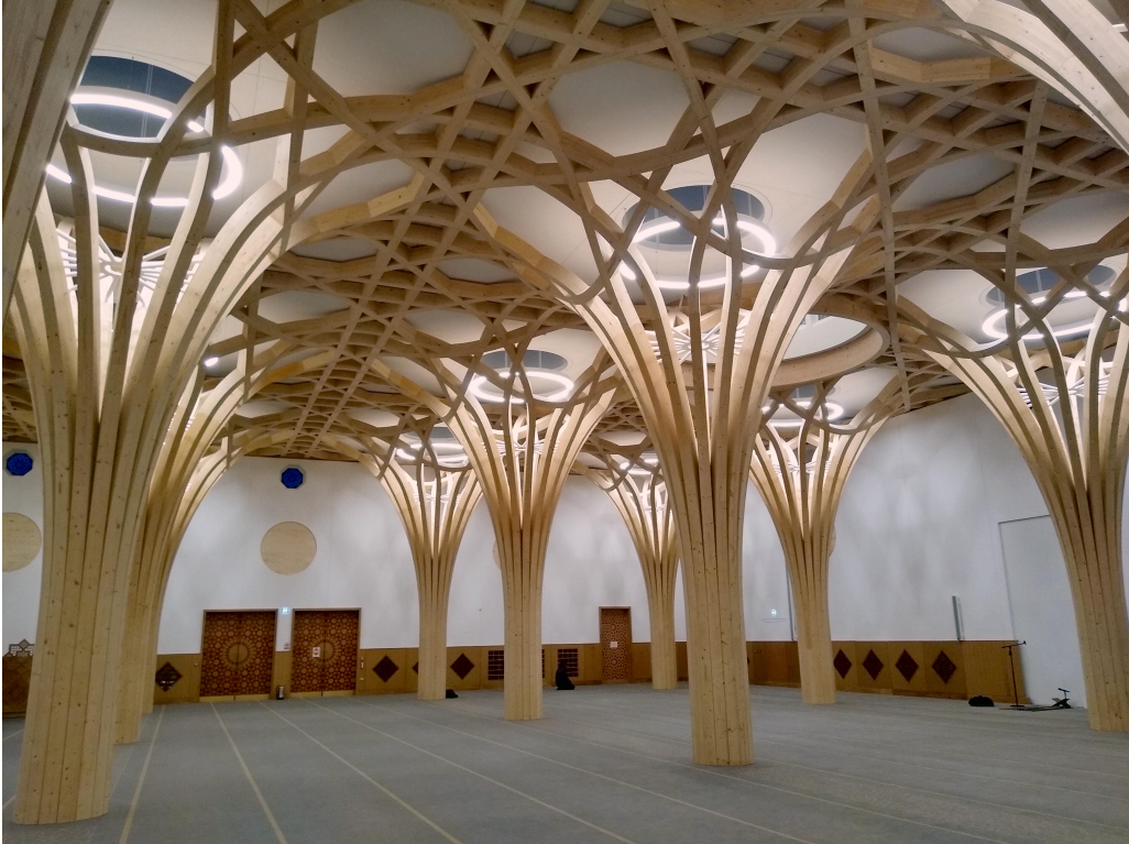
Figure 2.26: The roof at Cambridge Mosque consisting of a complex free-form timber framework, composed of single and double curved glulam beams. Team: Marks Barfield Architects, SJB Kempter Fitze AG, Blumer Lehmann and Design-to-Production
