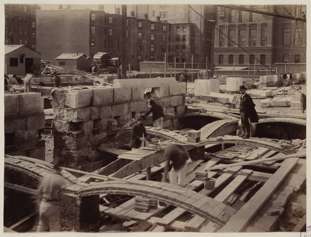
Figure 2.19: Master builder Rafael Guastavino standing on a recently finished arch during the construction of the Boston Public Library, 1889
