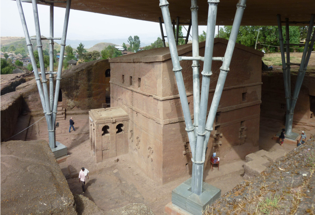
Figure 2.21: Temporary roof structures over the Biete Mariam Rock Church in Lalibela, Ethiopia, funded by the European Union
