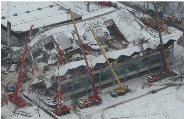
Figure 4. The Bad Reichenhall Ice Arena collapse (Photo credits ©LKA Bayern)
