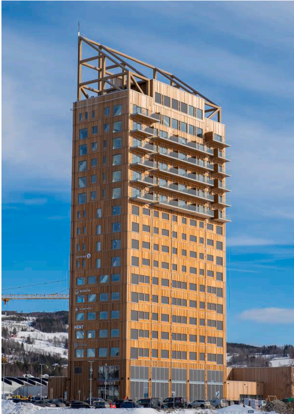
Figure 1. Mjøstårnet, the world's tallest timber building to date (Photo credits ©Moelven)
