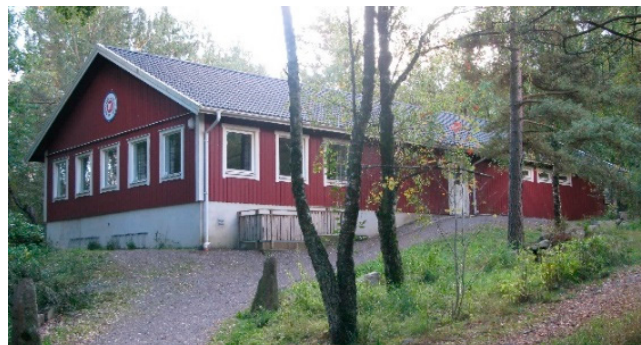
Figure 1. Image of the clubhouse building.
