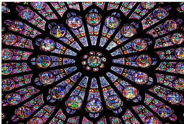
Figure 4.3: Medieval application of localized surface plasmon resonance. Light in certain wavelength intervals is absorbed and scattered by metal nanoparticles in the glass, producing colorful results. Notre-Dame de Paris.
