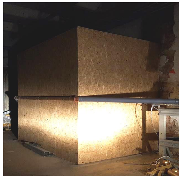
Fig. 2. Small test room inside the building.
