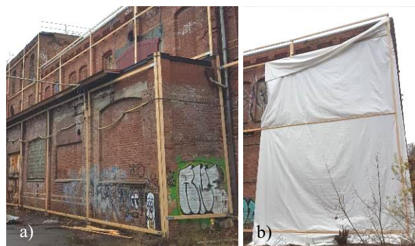
Fig. 8. (a) Exterior of the building prepared to be covered in plastic wrapping. (b) Part of the building covered in plastic, from November 2019.
